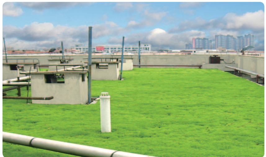
Green roof at ELPs production building
