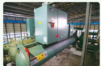
Magnetic Bearing Chillers
